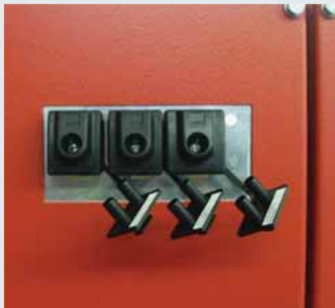
Passive DEHNcap/P voltage indicator used for an encapsulated switchgear installation.
