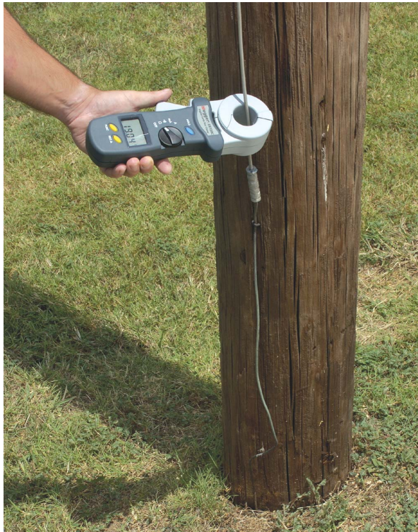
The DET20C instrument is shown being used to test a pole ground.
