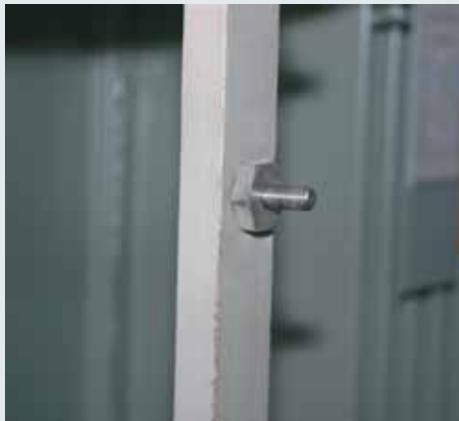
Earth connector with M12 threaded bolt for connection to an earthed part of the installation.
