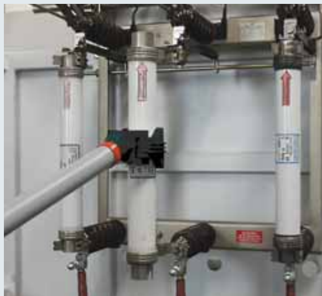
Angled (20°) SZ fuse tong for inserting and removing h.v.h.b.c. fuses.
