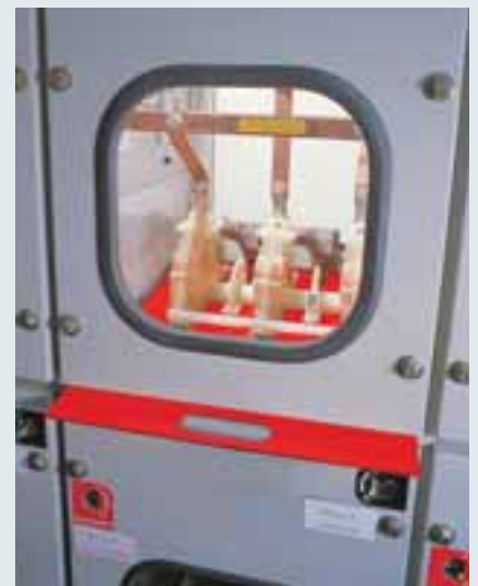
Inserting an insulating protective shutter, type A4.
