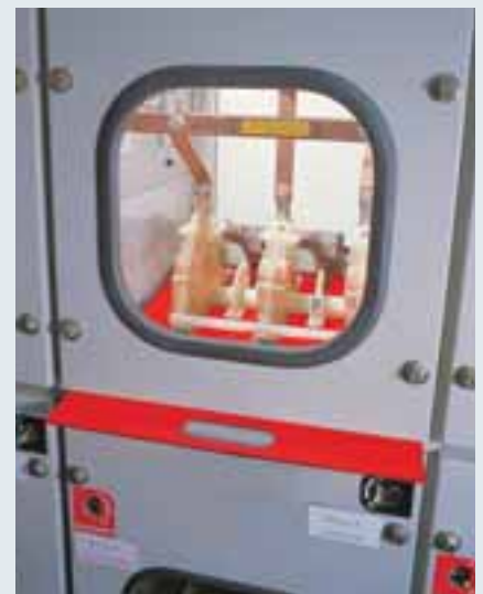
Inserting an insulating protective shutter, type A4.
