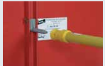
Operating rod with T pin shaft (bayonet type) and coupling with T pin shaft at the insulating protective shutter.
