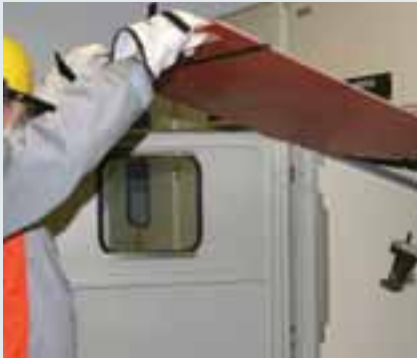
Inserting an insulating protective shutter, type A1, by hand.
