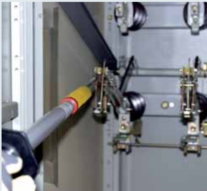
IS STK insulating rod with STK switching rod head used as switching rod.
