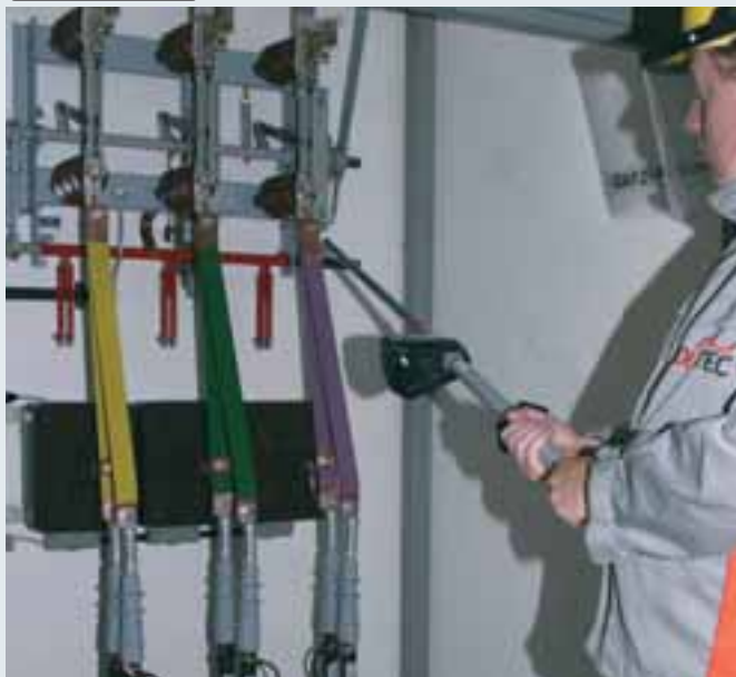
PHE voltage detector with visual indicator.
