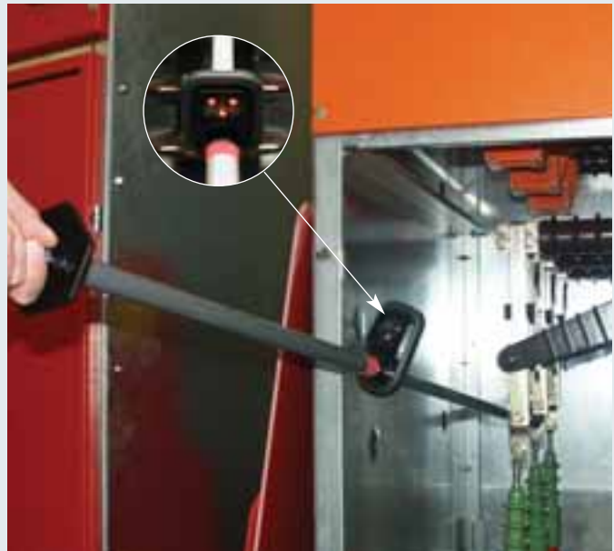
PHG II voltage detector used for a type-tested switchgear installation.
