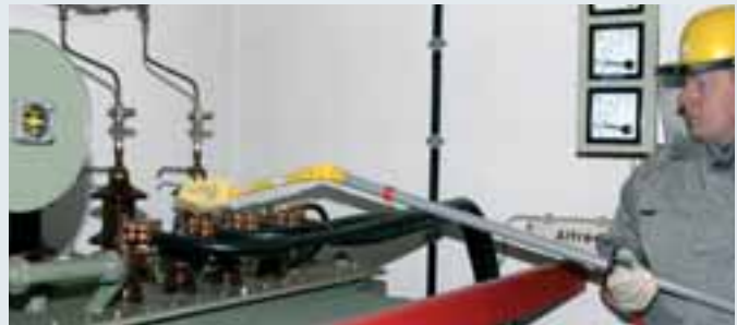
Dry and damp cleaning of a transformer under live conditions using the TFRS MS combined cleaning kit.
