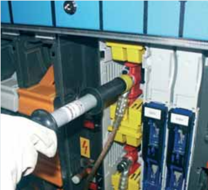
Installation of the the partly insulated earthing and short-circuiting device using earthing handle Type TI
