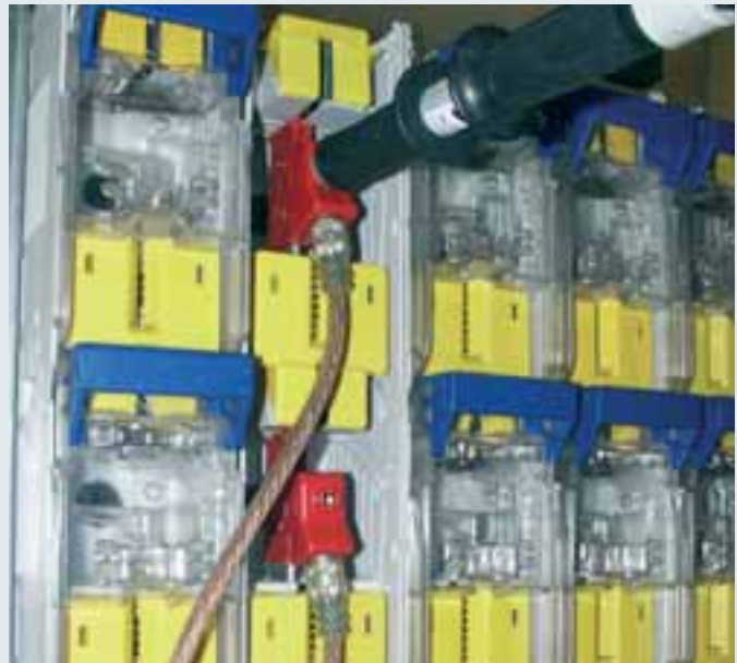
Installation of the fully insulated earthing and short-circuiting device using earthing handle Type VI.
