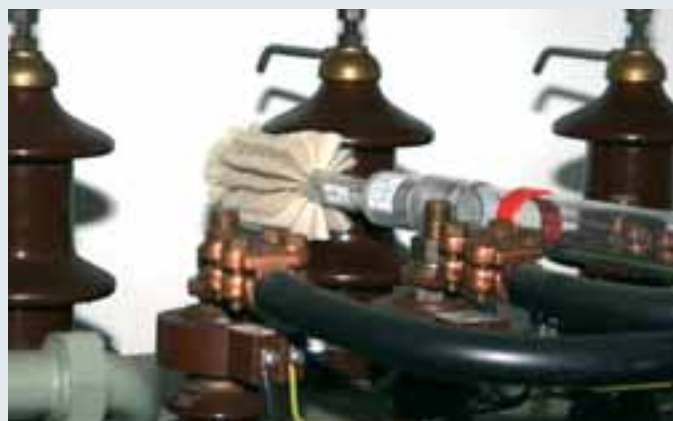
Cleaning an insulator with a tubular brush.
