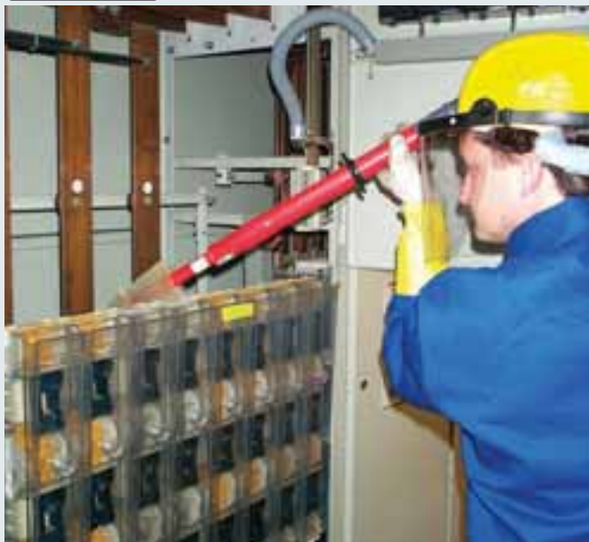
Live cleaning of a low-voltage switchgear installation using the TRS NS dry cleaning kit
